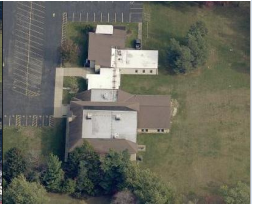
West Side View
